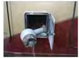
Dump Station Connector
